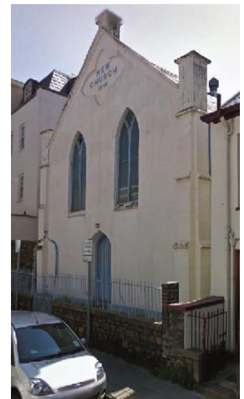
New Church, Jersey Google Street View
